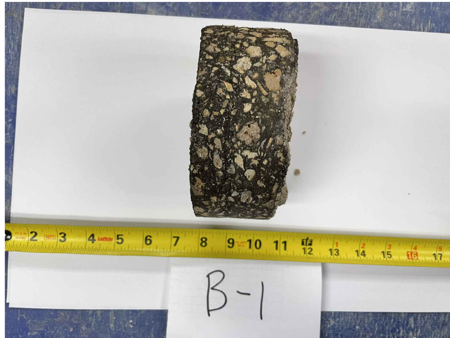
B-1: 2.25 INCHES THICK ASPHALT
